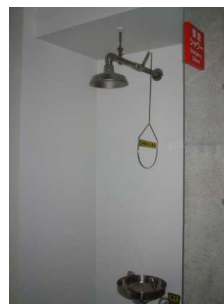
Emergency shower (wall-hanging type) : Pull the chain for a rinse. The shower will stop automatically.
