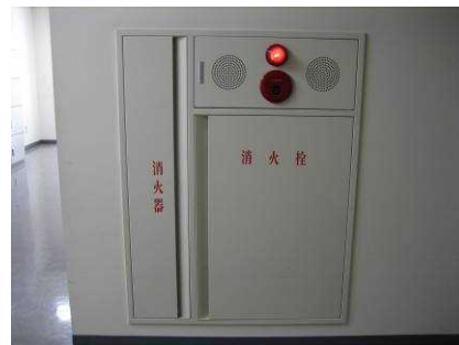
Fire alarm (top) and hydrant (bottom)
