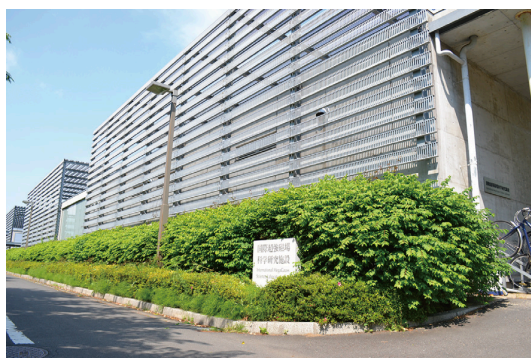
Fig. 1. The building C of the IMGSL.
