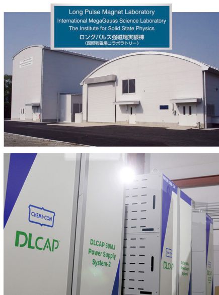
Fig. 2. Upper: The K-building for the supercapacitor power supply (left-hand side) and a long pulse magnet station (right-hand side). Lower: The supercapacitors have a total accumulation energy of 150 MJ installed in 2023 and are planned to drive the long pulse 60 T magnet and the first stage of the dual-coil 100 T non-destructive magnet.
