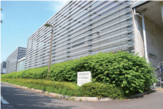
Fig. 1. The building C of the IMGSL.
