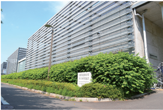
Fig. 1. The building C of the IMGSL.
