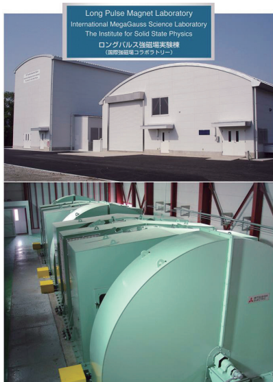
Fig. 2. Upper: The K-building for the flywheel generator (left-hand side) and a long pulse magnet station (right-hand side). Lower: The flywheel giant DC generator which is 350 tons in weight and 5 m high (bottom). The generator, capable of a 51 MW output power with the 210 MJ energy storage, is planned to energize the long pulse magnet generating 100 T without destruction.
