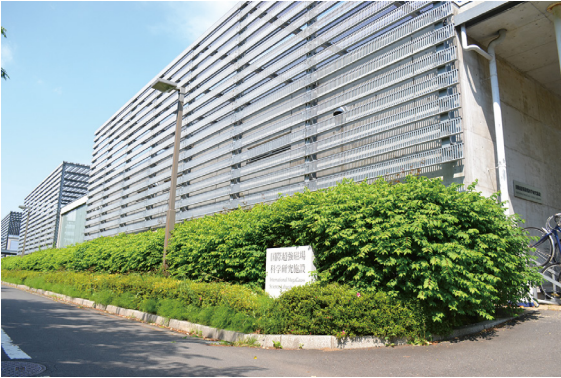
Fig. 1. The building C of the IMGSL.
