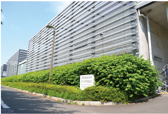
Fig. 1. The building C of the IMGSL.
