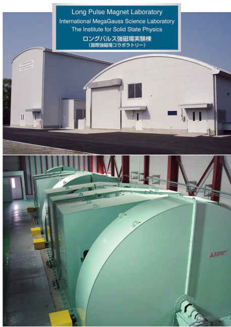
Fig. 2. The building for the flywheel generator (left hand side) and a long pulse magnet station (right hand side). The flywheel giant DC generator is 350 ton in weight and 5 m high (bottom). The generator, capable of a 51 MW output power with the 210 MJ energy storage, is planned to energize the long pulse magnet generating 100 T without destruction.
