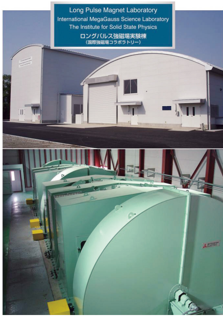
Fig. 2. The building for the flywheel generator (left hand side) and a long pulse magnet station (right hand side). The flywheel giant DC generator is 350 ton in weight and 5 m high (bottom). The generator, capable of a 51 MW output power with the energy storage 210 MJ, is planned to energize the long pulse magnet generating 100 T without destruction.
