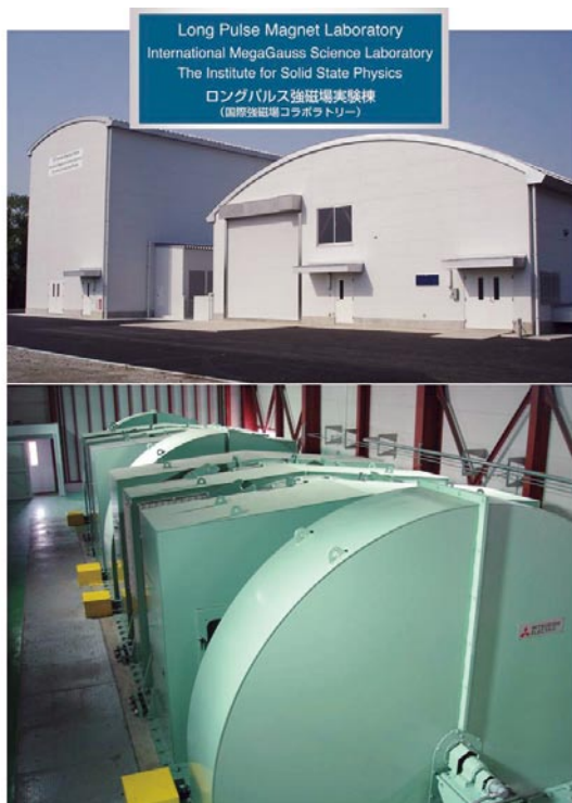
Fig. 1. The building for the flywheel generator (left hand side) and a long pulse magnet station (right hand side). The flywheel giant DC generator is 350 ton in weight and 5 m high (bottom). The generator, capable of a 51 mega watt out put power with a 210 mega joule energy storage, is planned to energize the long pulse magnet generating 100 Tesla without destruction.
