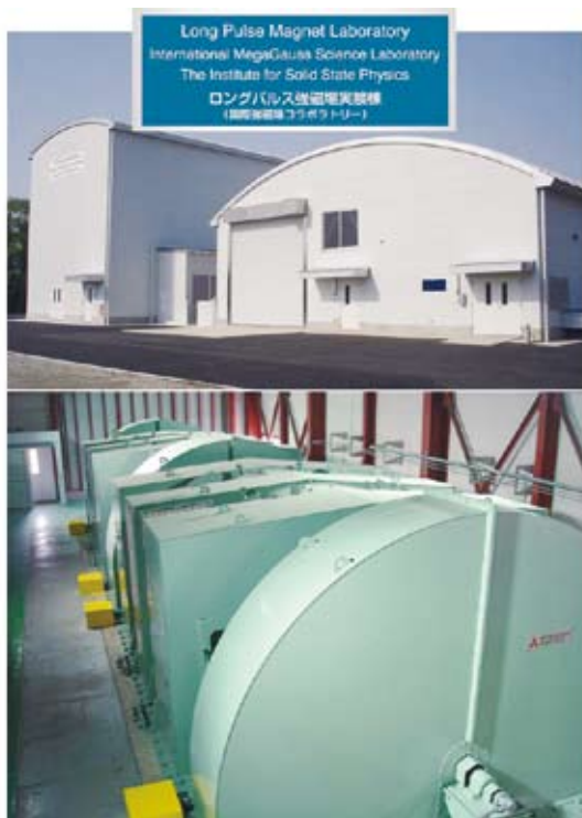
Fig. 1. The building for the flywheel generator (right hand side) and a long pulse magnet station (left hand side). The flywheel giant DC generator is 350 ton in weight and 5 m high (bottom). The generator, capable of a 51 mega watt out put power with a 210 mega joule energy storage, is planned to energize the long pulse magnet generating 100 Tesla without destruction.
