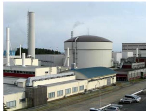
Fig. 1. The reactor hall of JRR-3. The eight neutron scattering instruments are attached to the horizontal beam tubes in the reactor experimental hall. Two thermal and three cold guides are extracted from the reactor core towards the guide hall located to the left.
