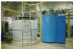
⑪液体ヘリウム貯槽 (左) STATEBORN社製 6,000L 蒸発率 1.0%/day
