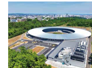
放射光施設 Synchrotron radiation facility
