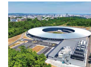
放射光施設 Synchrotron radiation facility
