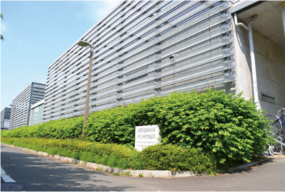
Fig. 1. The building C of the IMGSL.
