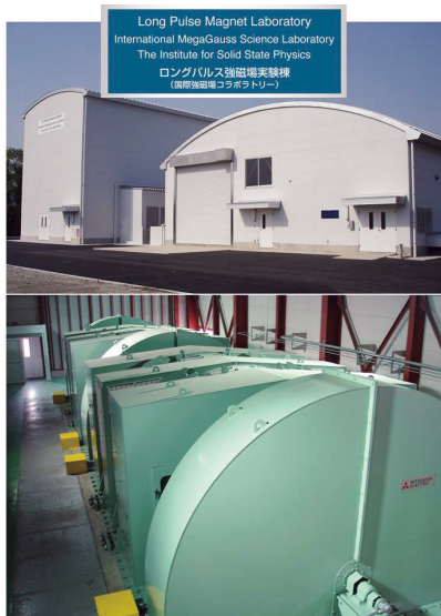
Fig. 2. Upper: The K-building for the flywheel generator (left hand side) and a long pulse magnet station (right hand side). Lower: The flywheel giant DC generator which is 350 ton in weight and 5 m high (bottom). The generator, capable of a 51 MW output power with the 210 MJ energy storage, is planned to energize the long pulse magnet generating 100 T without destruction.
