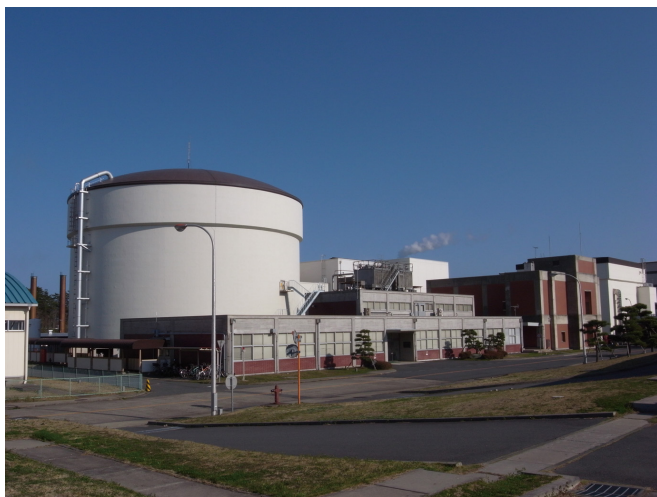
Fig. 1. The reactor of JRR-3. The eight neutron scattering instruments are attached to the horizontal beam tubes in the reactor experimental hall. Two thermal and three cold guides are extracted from the reactor core towards the guide hall located to the left.
